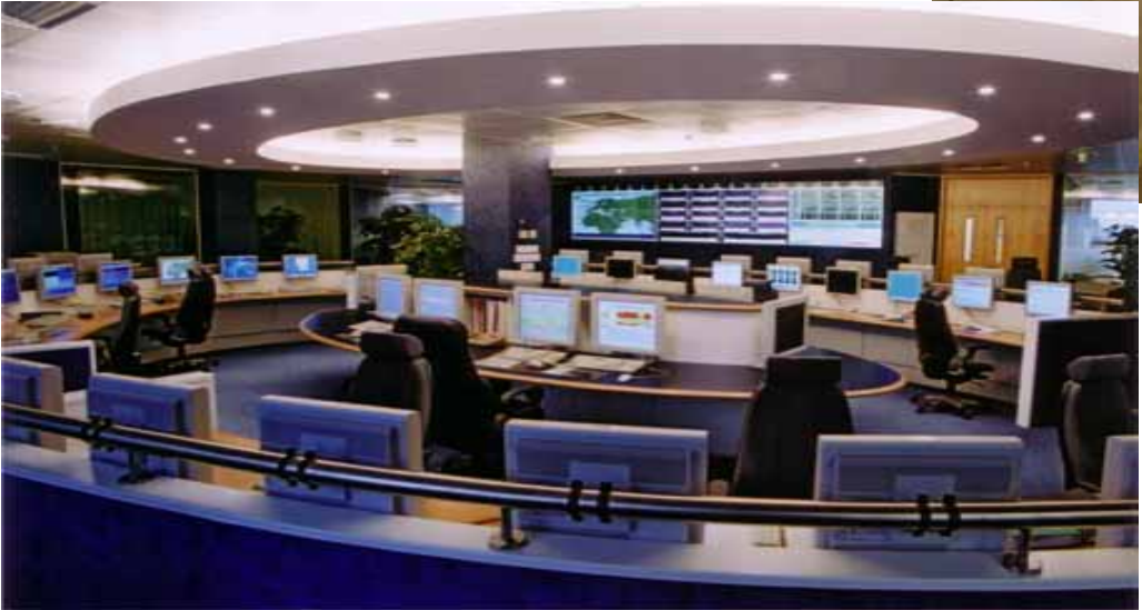
Network Operations Centre
